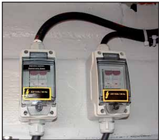
AUTOMATIC BREAKERS OF THE SHORE POWER SOCKETS
