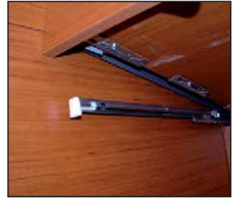
REMOVING THE DRAWER LEVER + RAILS
