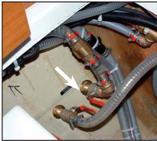
WATER INLET VALVE OF THE GENERATOR
