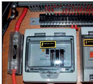
CONSUMING APPLIANCES CIRCUIT BREAKERS
