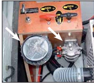
WATER FILTER + FUEL FILTER OF THE GENERATOR
